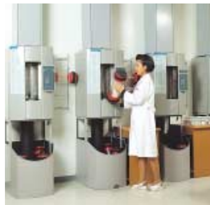
Pneumatic Tube System
