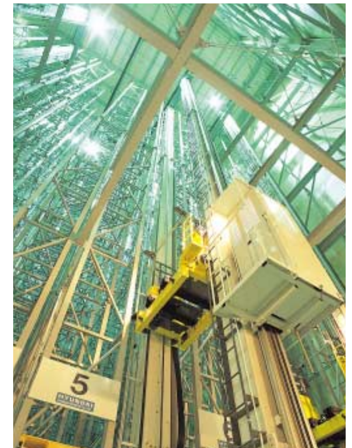
High Rised Automatic Warehouse
