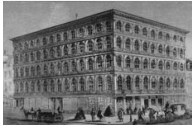
E.V. Haughwout & Company store at Broadway and Broome Street in New York City, site of the world's first passenger safety elevator.
