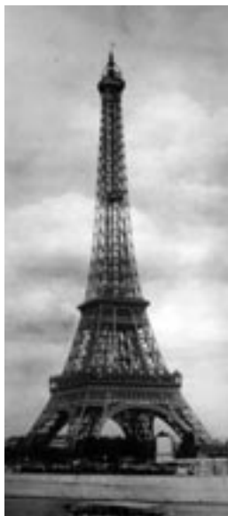
An engineering marvel of its day, the Eiffel Tower rose to a height of 300 meters (984 ft), served by elevators operating at a rate of more than 2 meters (6.5 ft) per second.
